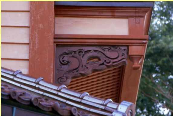
Second-floor veranda supports
