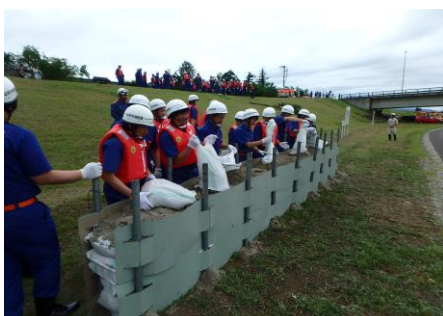
"土留鋼板工法状況、"
